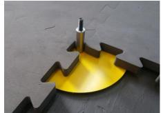
**<u>Step 4-5 Optional</u>**: In order to allow the bolt to extend through the tile, trim the small corner extension on the fourth tile. Place that tile at the intersection.
